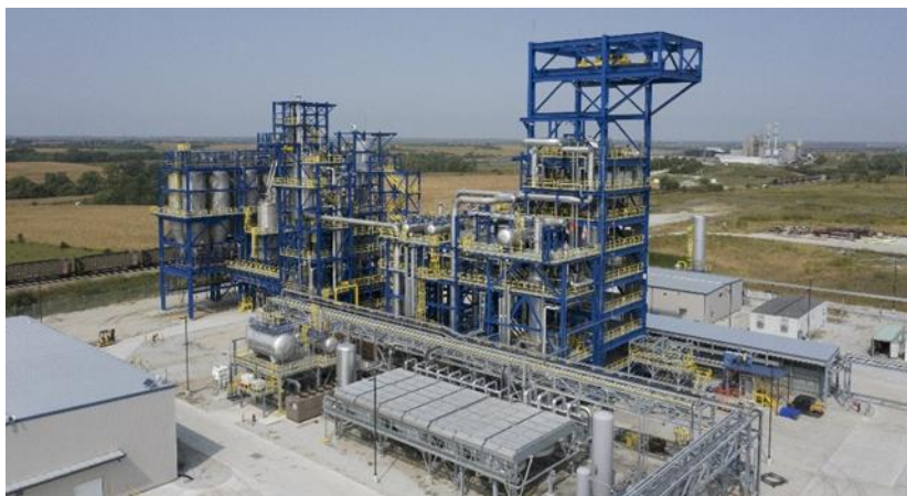
Figure 9 – Monolith’s emissions free hydrogen plant [23]
